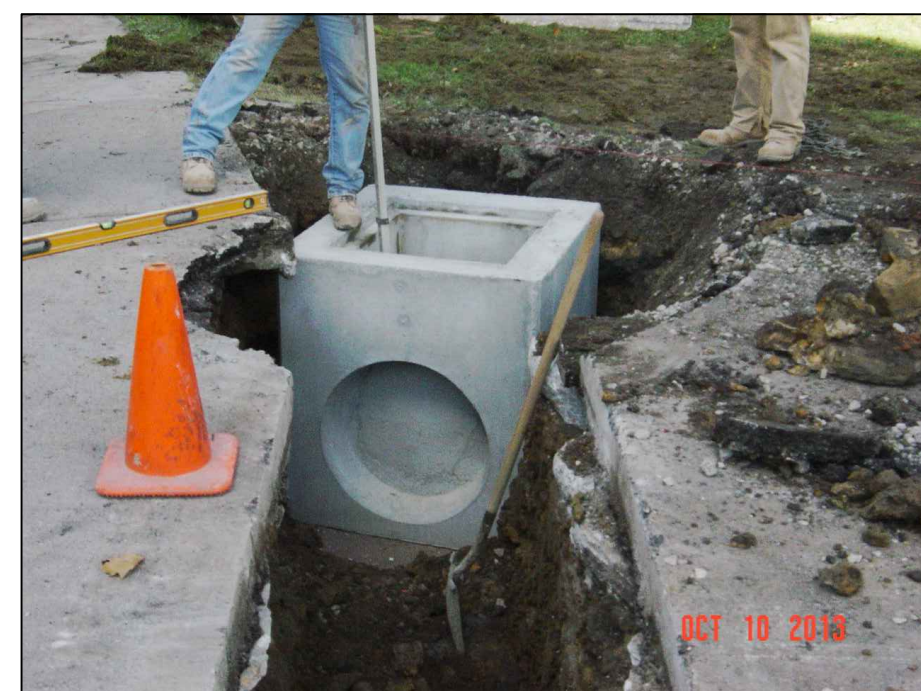
Drop Inlet at Handicapped Parking Spot
