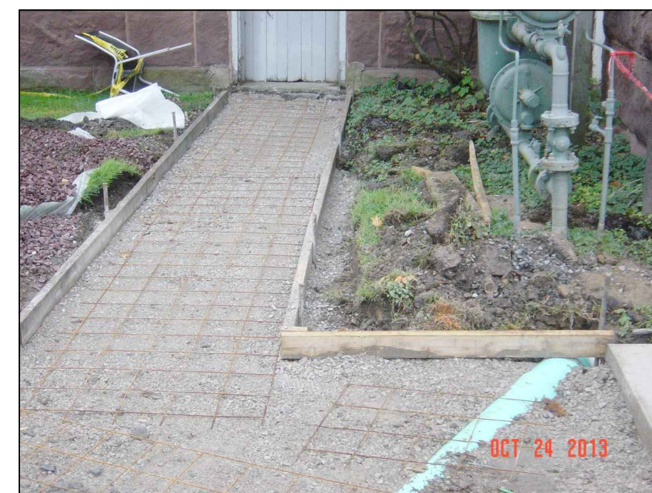
Downspout Pipe Conduit at Northwest Corner
