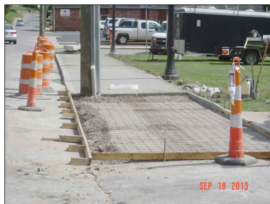
Sidewalk along Walnut Street by Electric Pole
