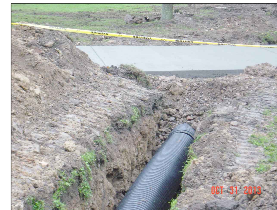
Storm Sewer Construction toward Church Street
