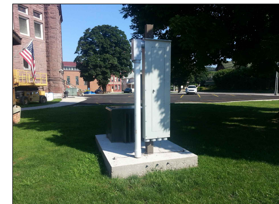
New Electric Connection and Completed Parking Area
