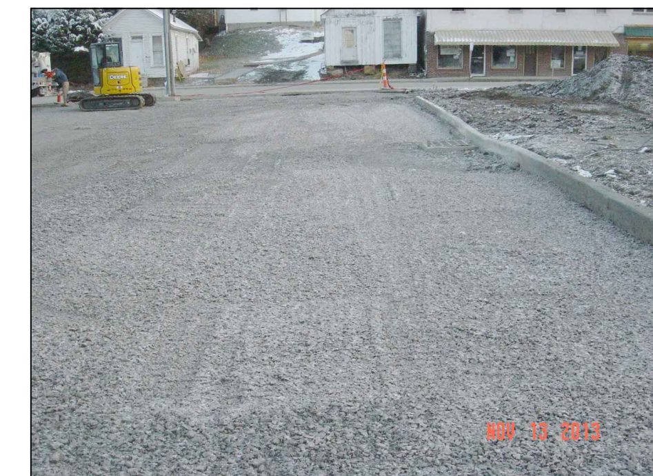
Parking Area Rock Subbase prior to Asphalt
