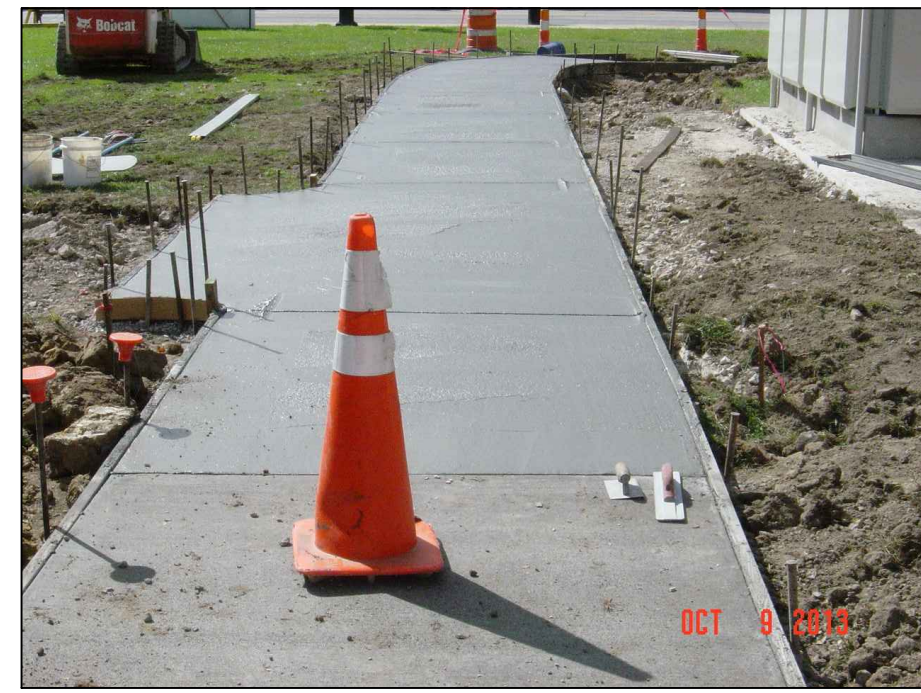
Gazebo Conduit at Rebars with Red Ribbons
