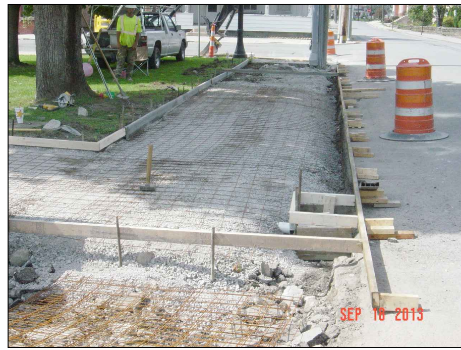
Walnut St Looking NW with Dumpster Pad and Drop Inlet
