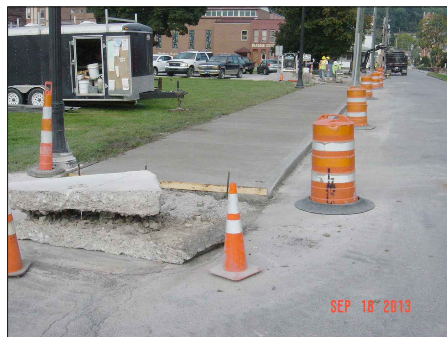
Sidewalk along Walnut Street
