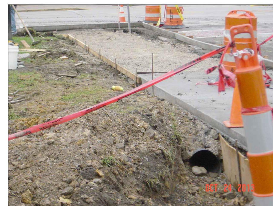
Storm Sewer under Sidewalk at Church Street
