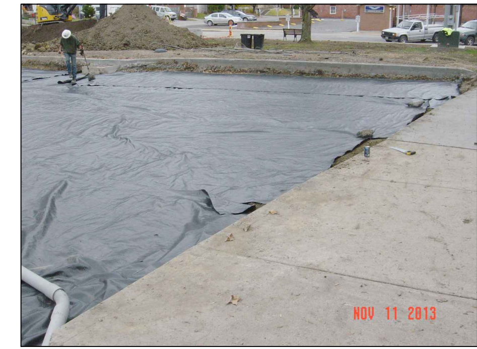
Fiber Optic Conduit and Filter Fabric under Parking Area
