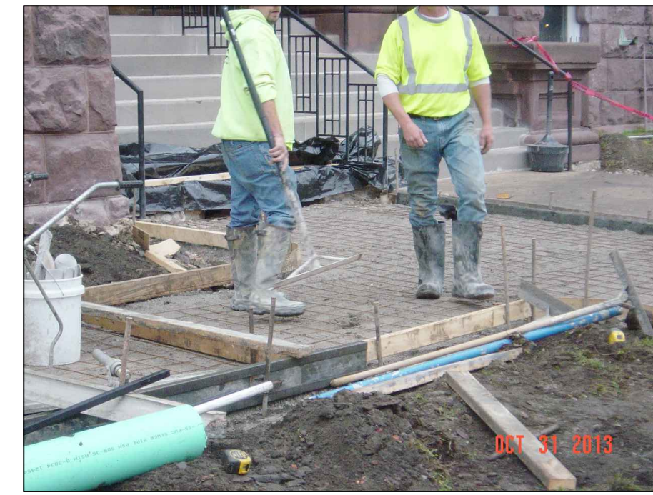
Sidewalk at Court House Front Steps
