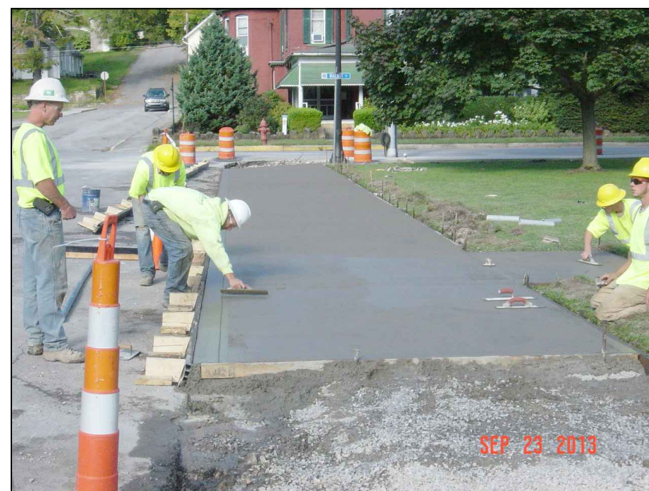
Sidewalk Construction along Church Street
