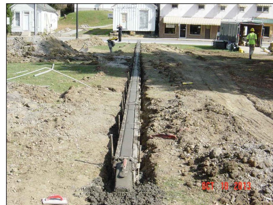
Curb Construction at Southern End of Parking Area
