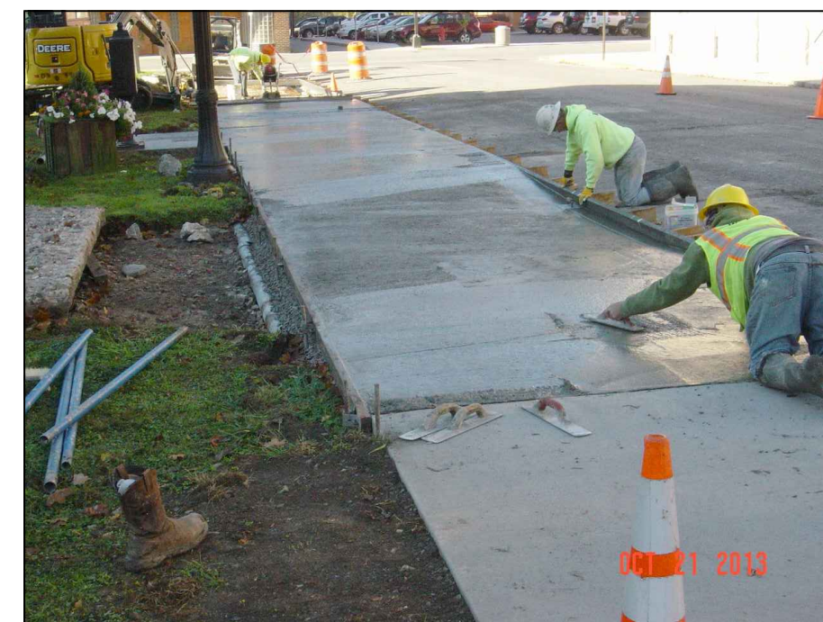
Handicapped Ramp Construction on Church Street
