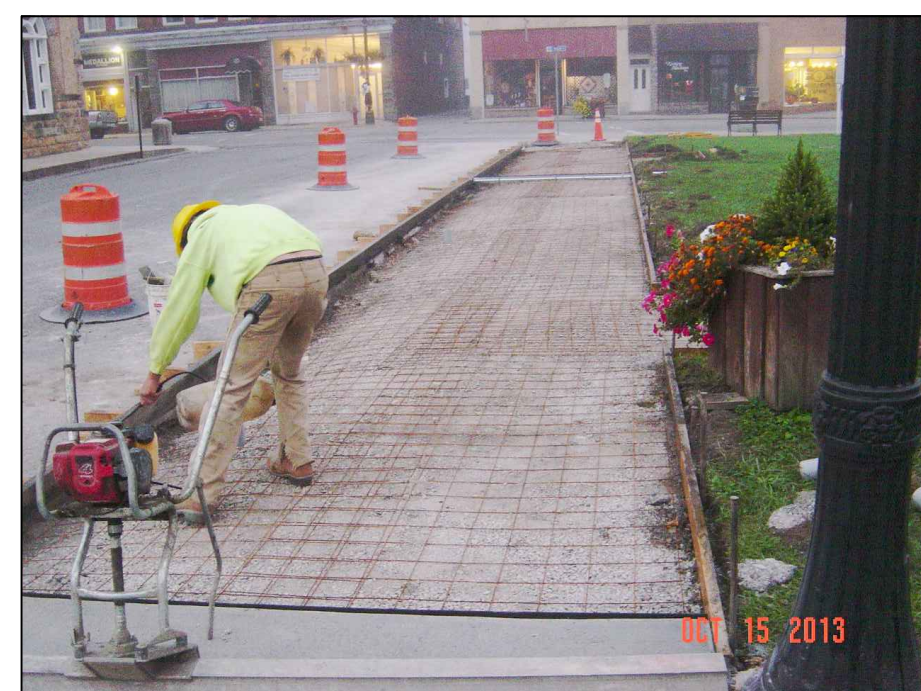
Sidewalk Construction on Court Street
