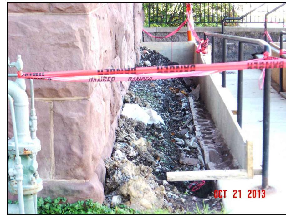
Handicapped Ramp Wall Reconstruction
